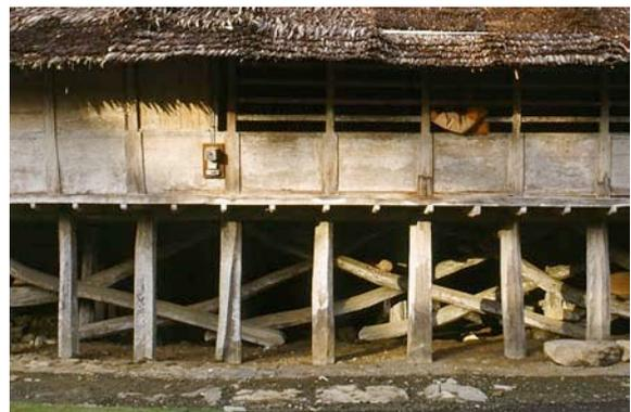
Fig. 4: Foundation of a building in North Nias
